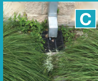
Downspout diverted into swale area through catchbasin and perforated pipe
