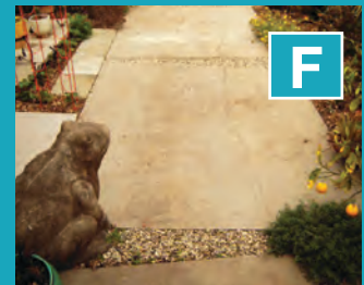
Horizontal 3"-6" cuts in walkway and driveway
