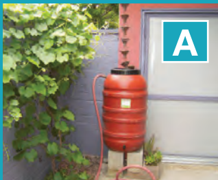
Rainbarrel with overflow into planter or permeable driveway
